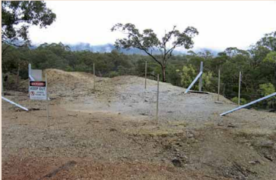
Fencing and signage was not a long-term management solution.
