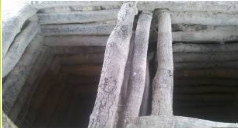
ASM Pits Supported using Cut Trees
